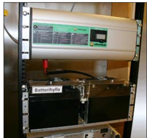
BAS 19" with battery shelf-mounted on 19" stand.
