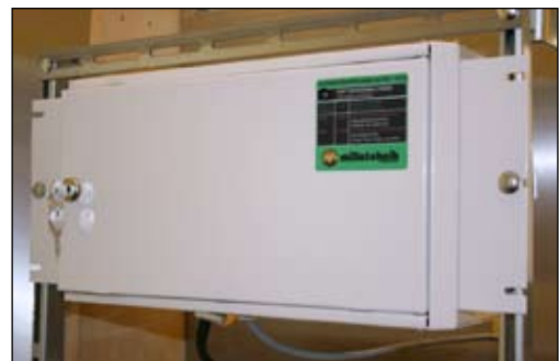
The ECO XS is installed on a 19" stand with the enclosed 19" angle brackets.
